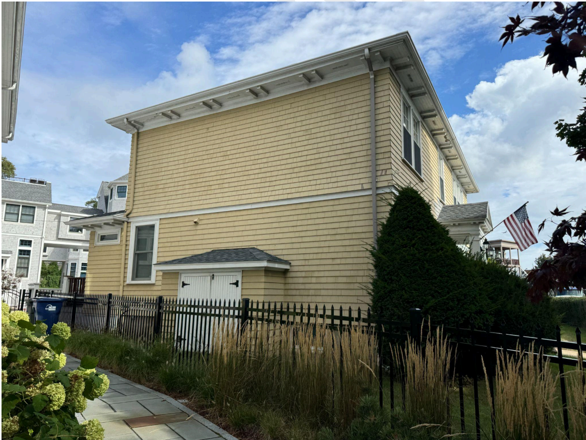
Figure 7: 1812 Columbia Road west facade, facing northeast. October 2, 2024.
