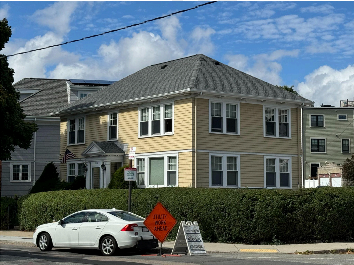
Figure 3: 1812 Columbia Road, facing northwest.
