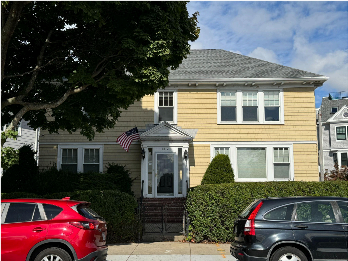
Figure 1: 1812 Columbia Road, facing north (northwest). October 2, 2024.
