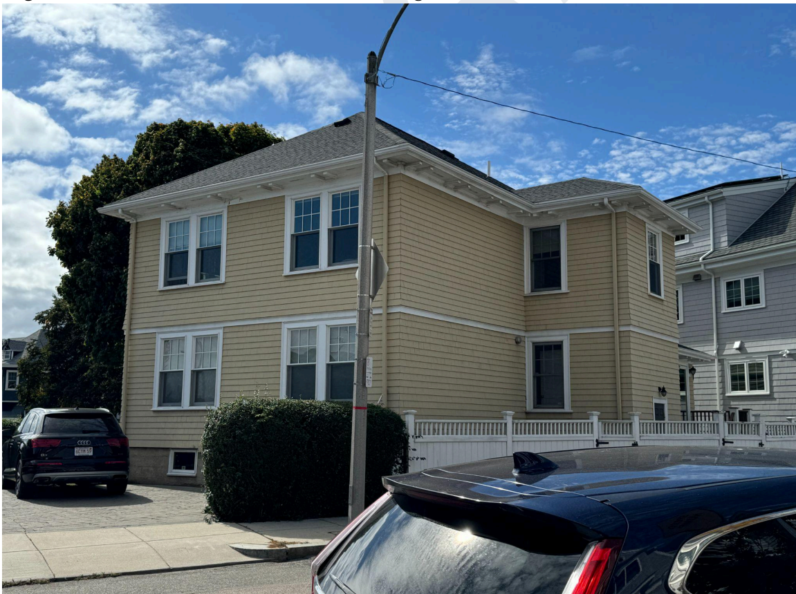
Figure 5: 1812 Columbia Road east and north (partial) facades, facing southwest. October 2, 2024.
