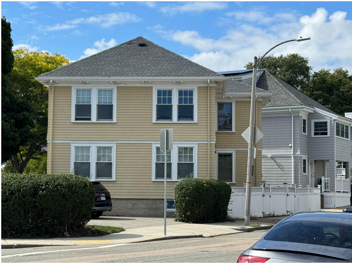
Figure 4: 1812 Columbia Road, east facade, facing west. October 2, 2024.
